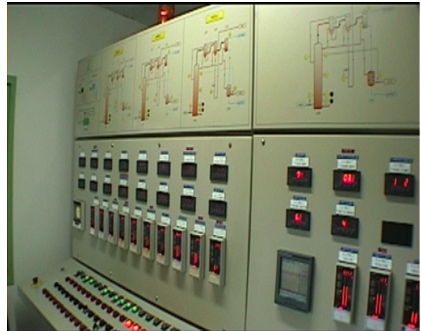
Automated control console of the distillation columns of the Simon distillery. Photo: Y.-M. Richer.
